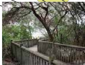
ADA RAMP / BOARDWALK
