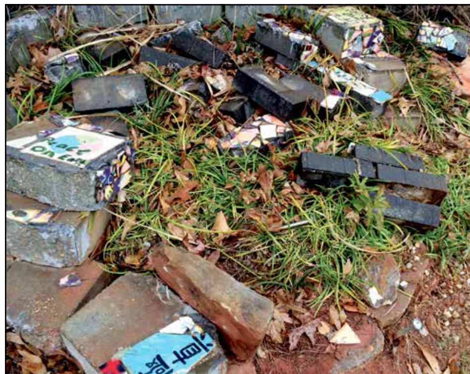
The Peace Garden as demolished, January 2017
