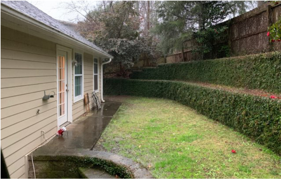
Back of house and retaining wall
