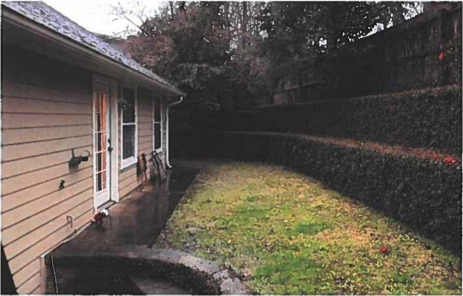
Back of house and retaining wall
