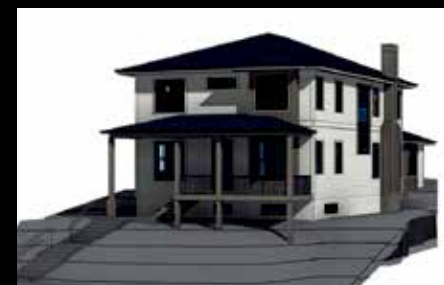
25 Lakeview Road New Construction – Kirkwood
