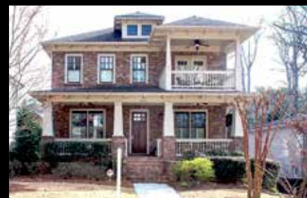
1595 Marlbrook Drive Coming Soon — $1,315,000
