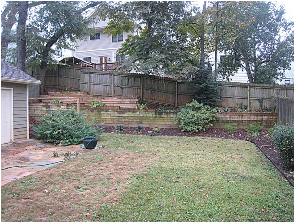
View toward back of lot with retaining walls and embankment
