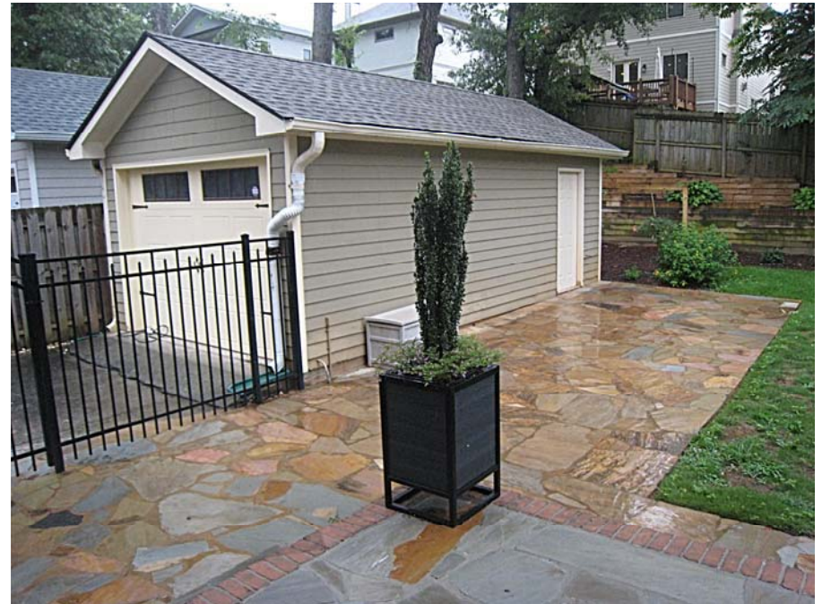
Existing stone patio to be removed
