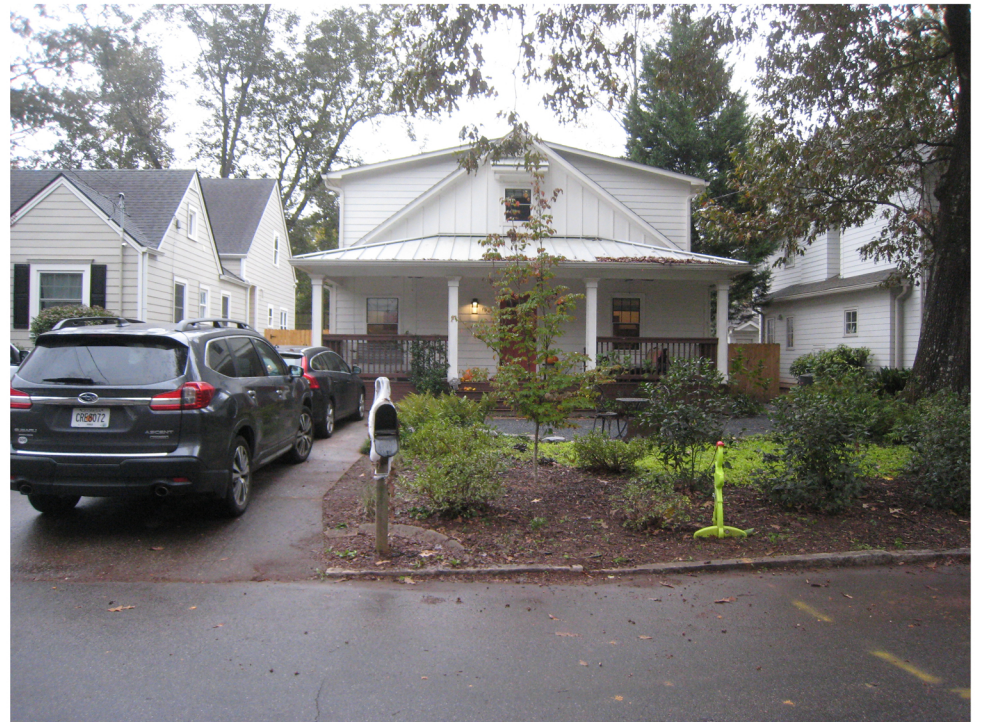
2057 - two houses to west (right)
