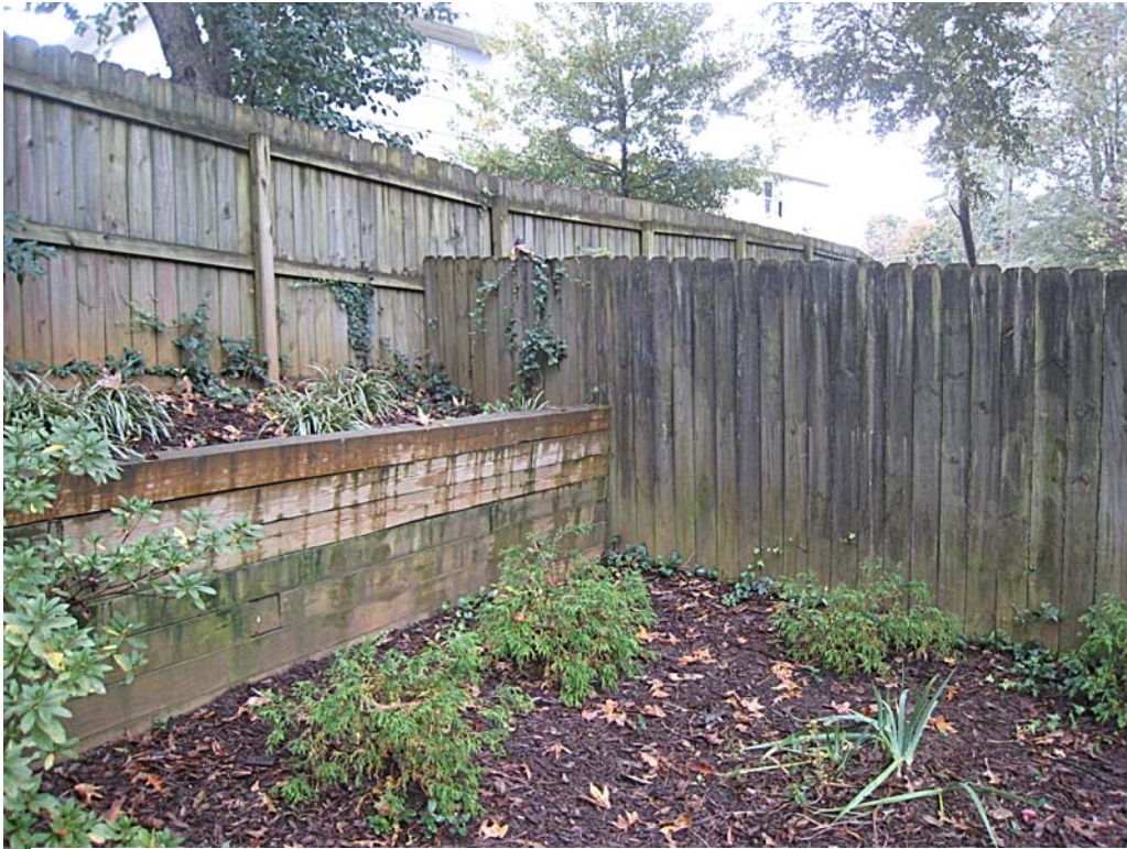
Existing retaining wall and fence at southwest corner of 2069
