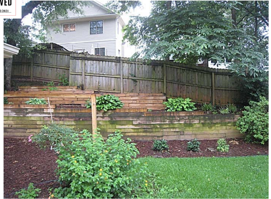
Existing retaining walls to remain
