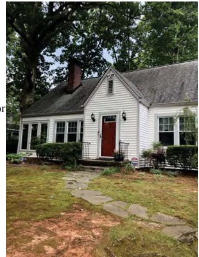
Existing front house entry
