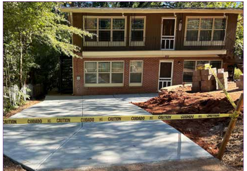
Walkway to Joe’s Place Repaved
