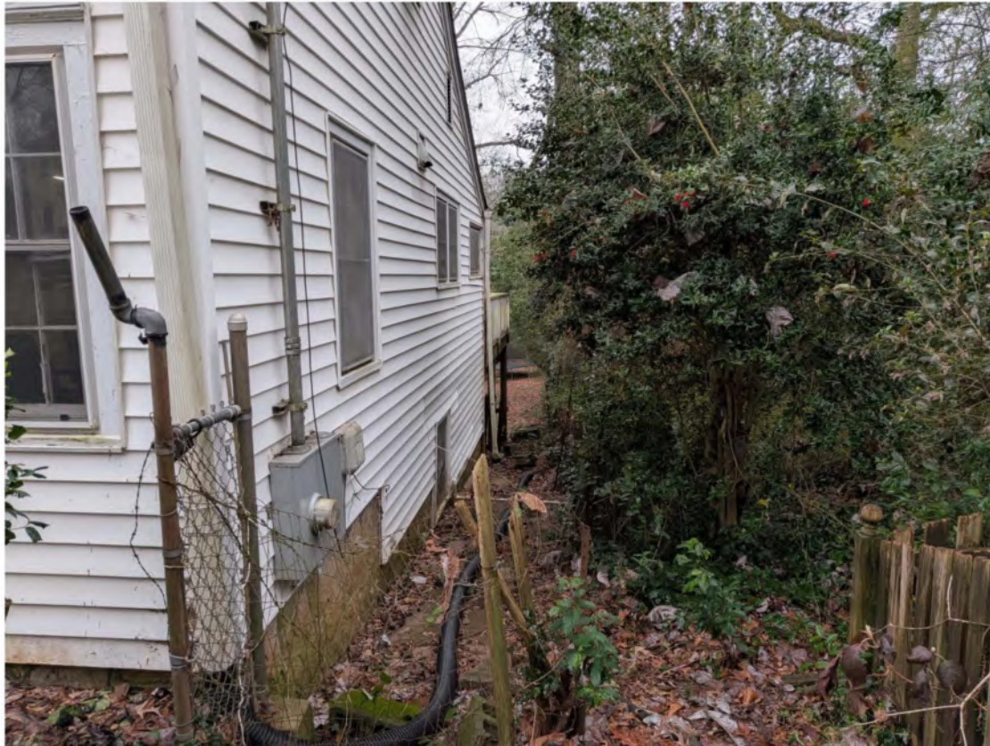
Western side of house
