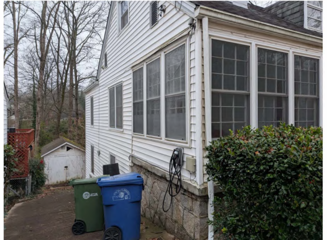
Eastern side of house
